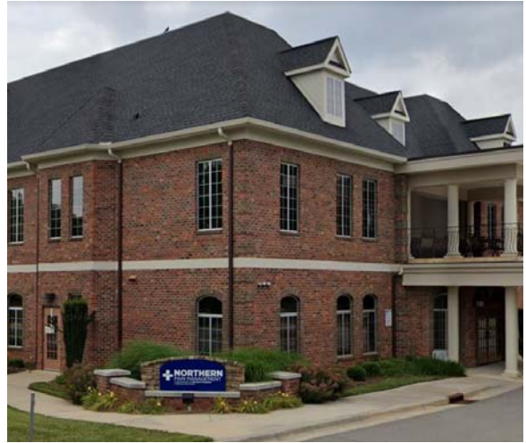
Figure 3.9 Example of Wall Materials
