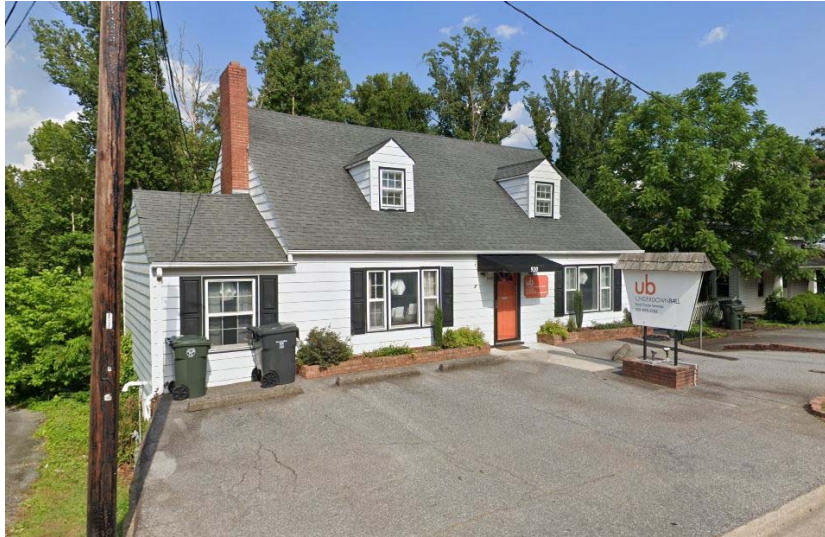
Figure 3.7 Example of a Primary Building Entrance
